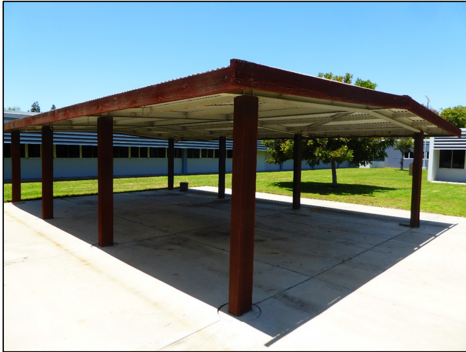
Photograph 4: Shade structure with eight support posts with added wood encasements, located in southwest courtyard of Building F; facing northwest, May 28, 2019.
