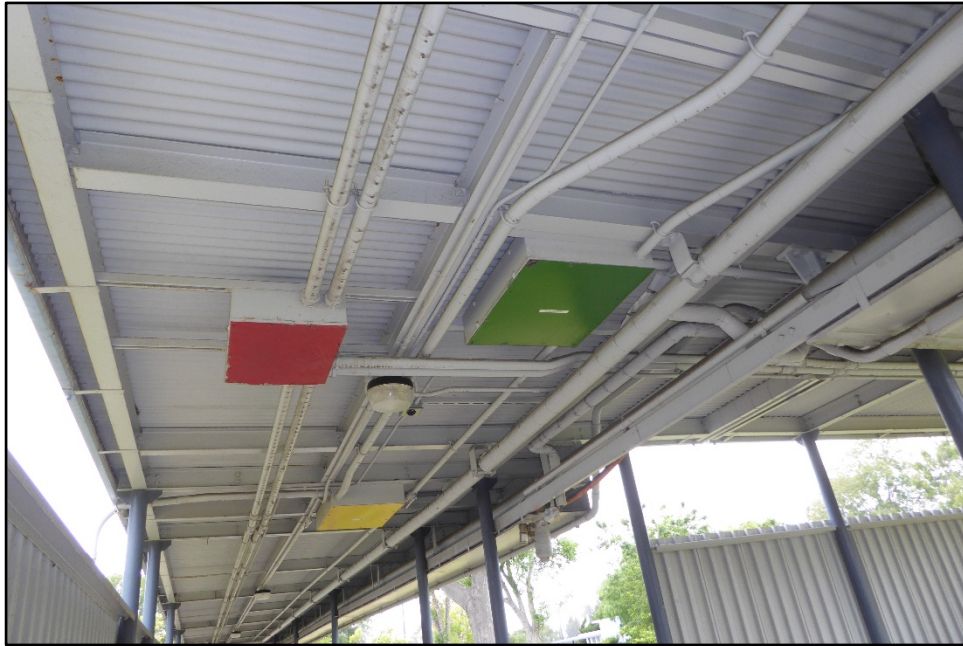
Photograph 4: Detail view of steam and utility distribution network carried via covered walkways; facing southwest, May 30, 2019.
