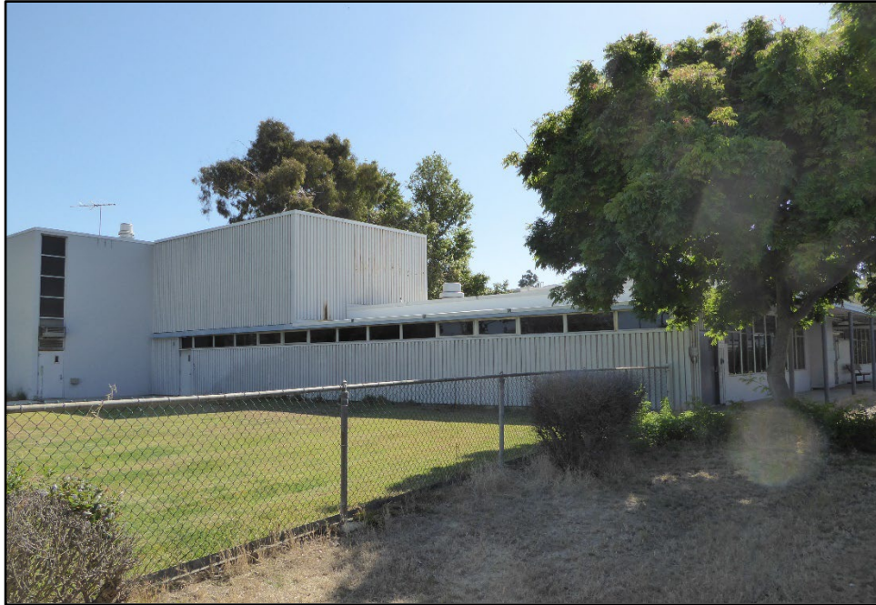
Photograph 2: Southwest corner of Residence 21-24 (Building K), showing wood-slat cladding; facing east / southeast, May 29, 2019.
