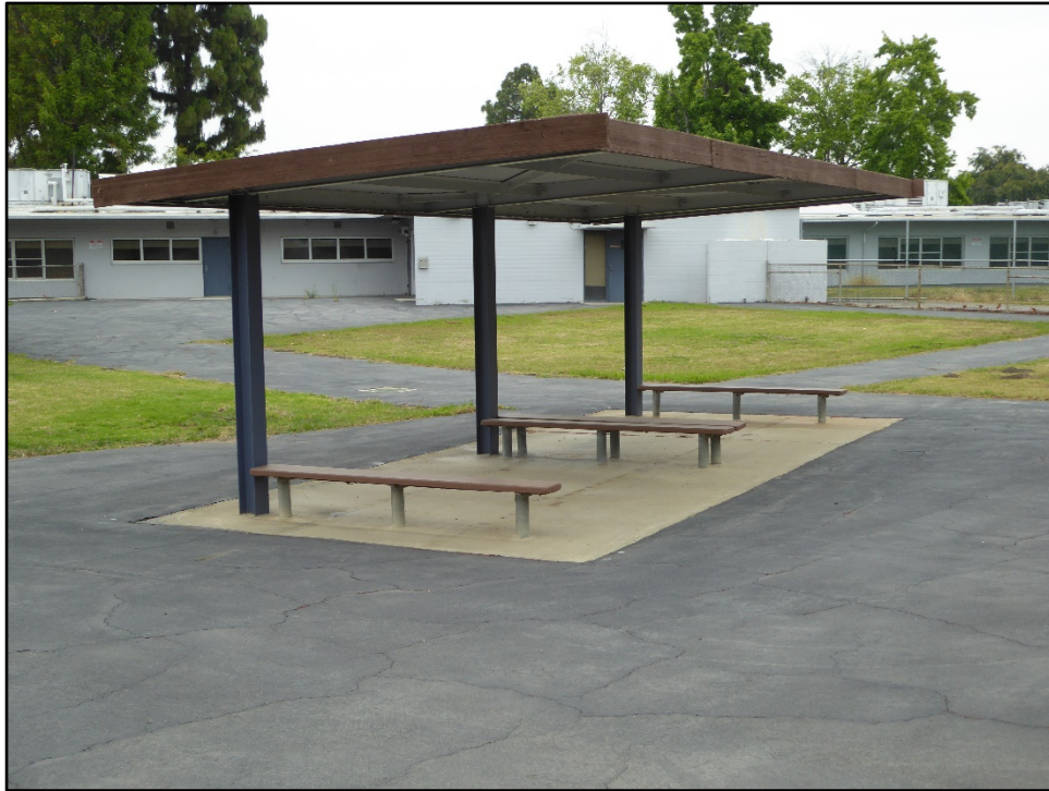
Photograph 6: Shade structure with three support posts with added wood encasement along roofing and three added fiberglass benches, located in southwest courtyard of Building B; facing northeast, May 29, 2019.
