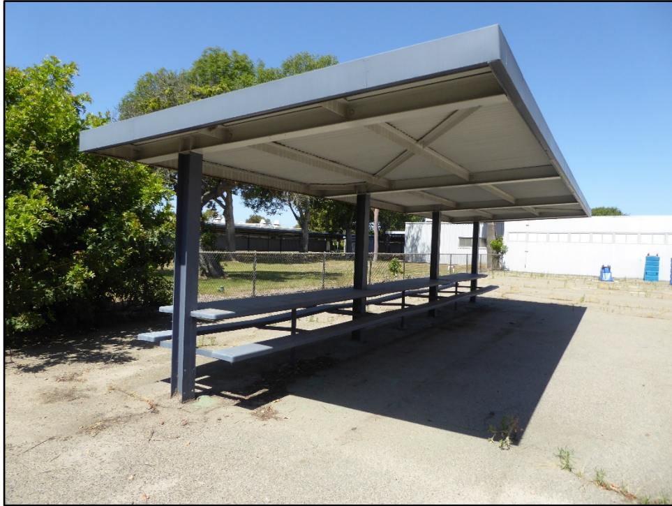
Photograph 2: Shade structure with four support posts and fiberglass bench and table, located in the east courtyard of Building P; facing southwest, May 28, 2019.
