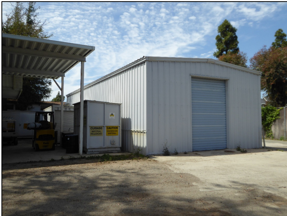
Photograph 12: Modern prefabricated Butler-type building, showing rear (northeast) shed-roof shade structure of automotive shop (left); facing north / northeast, May 29, 2019.
