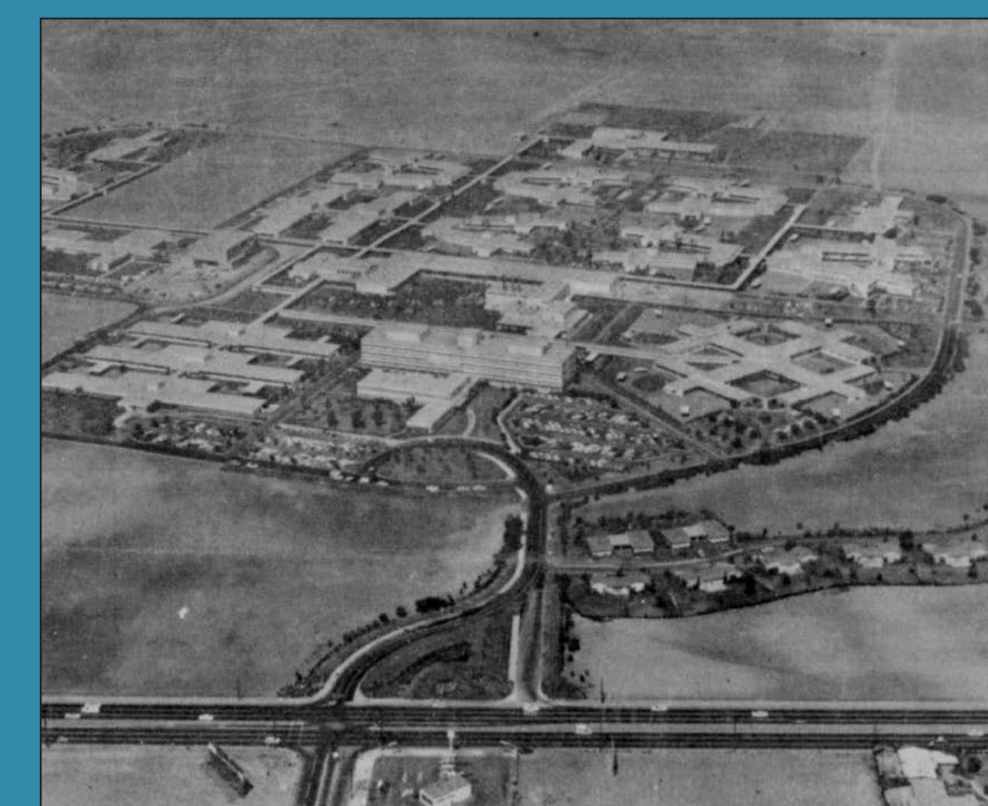
Fully developed Fairview State Hospital Main Campus in 1983. Source: Fairview: Costa Mesa State Hospital will have a New Name, from the Collections of the Costa Mesa Historical Society.
